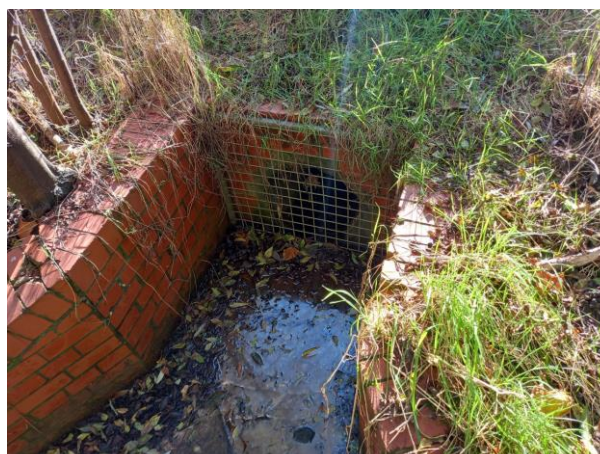
Photo 8: Outlet of culvert drain into basin
