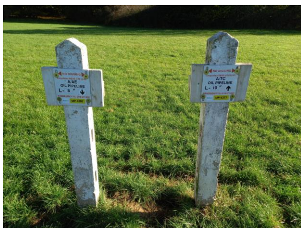
Photo 5: Surface location of oil pipes
