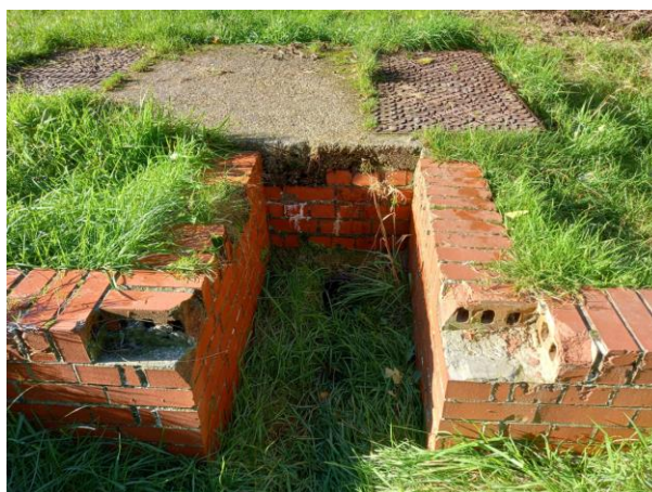
Photo 7: Culvert drain
